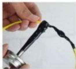
2. Apply liquid tape to wire
