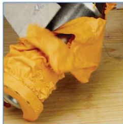
Remove paint on the surface of
