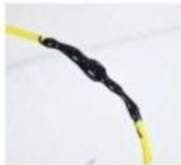
3. Place after application about 4 hours
