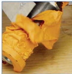
Remove paint on the surface of
