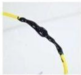
3. Place after application about 4 hours
