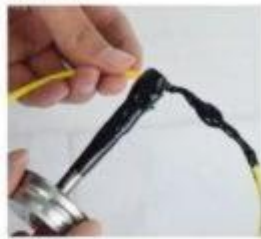
2. Apply liquid tape to wire
